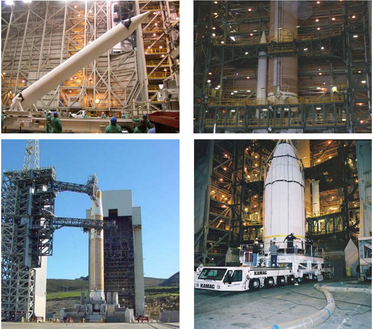
Figure 7. Solid rocket motor mounting, propellant tanking test, and encapsulated payload mate to vehicle.
