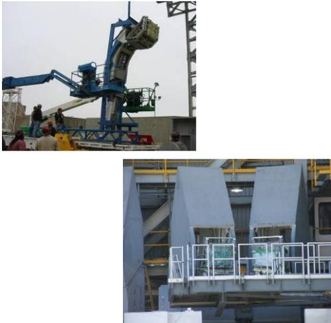
Fig. 8: Tail Service Mast (TSM) main structure and housing installation.
