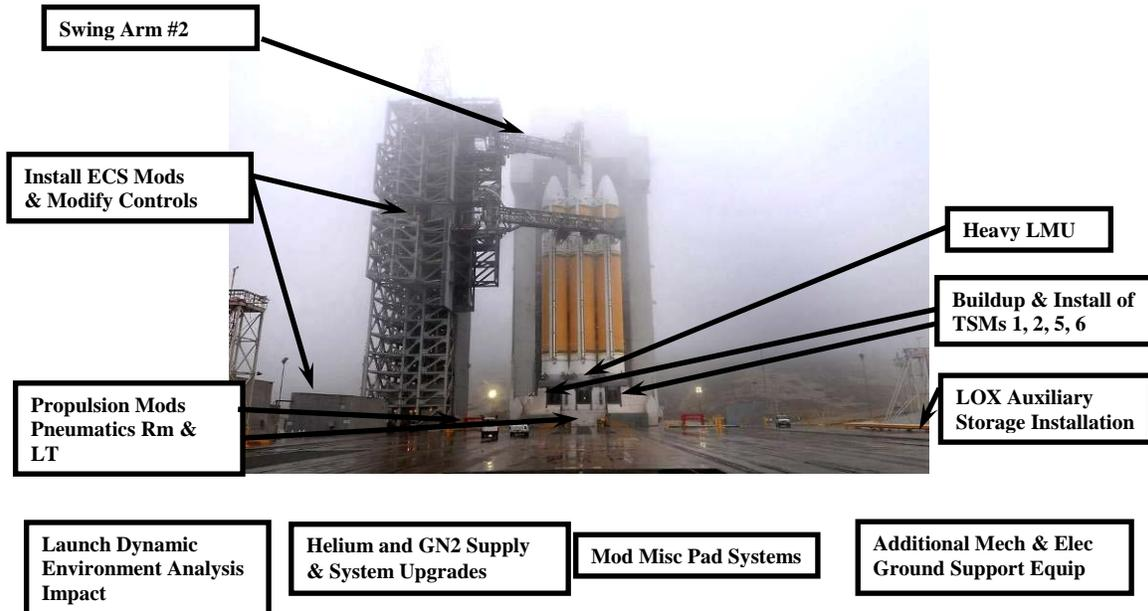
Fig. 7: SLC-6 Heavy Launch Vehicle (HLV) Modification Overview
