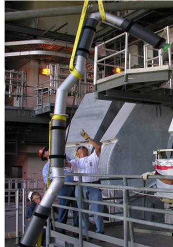
Fig. 9: Vacuum Jacketed Fill/Drain Line Installation
