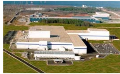
Figure 13. Delta Production Facility, Decatur Alabama, U.S.
