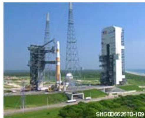
Figure 12. Launch Complex 37 at CCAFS.
